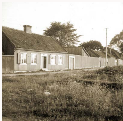
The Krusenstierna Gardens' utility buildings along Stora Dammgatan. The gardener's cottage in the foreground.
