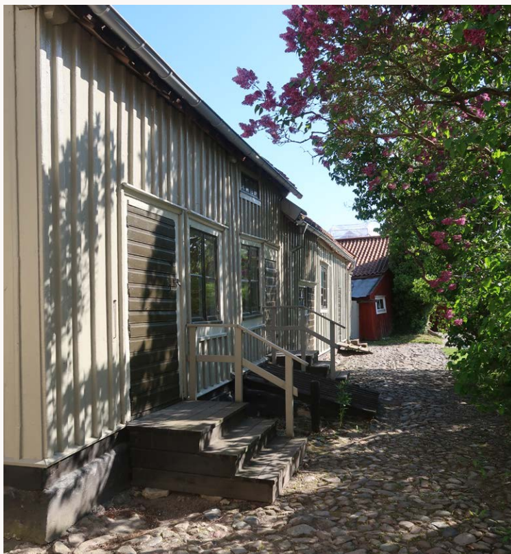
The row of utility buildings includes a brewhouse, farmhands' quarters, a woodshed, cowshed, latrine and henhouse. The barn and wagon house has been converted into a café.
